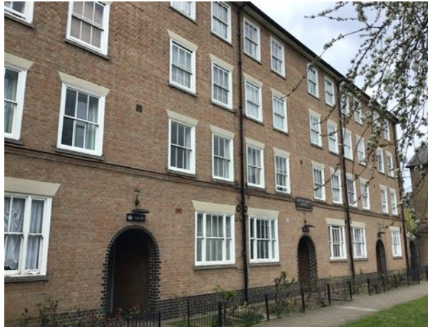
e.g. Barnersbury House, Holloway Estate
