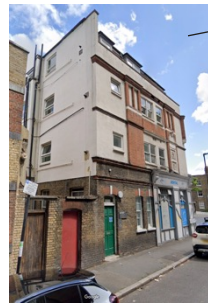
York House has a complex façade. Windows, ventilation and flat roof insulation could be priorities along with PV.
