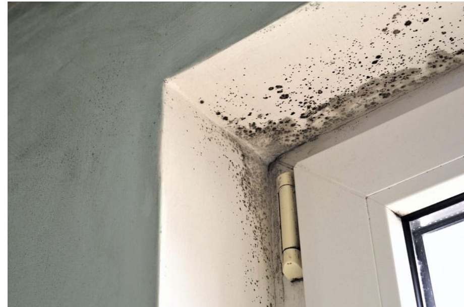
Cold bridges at junctions can be worse after a retrofit, leading to condensation and mould.
