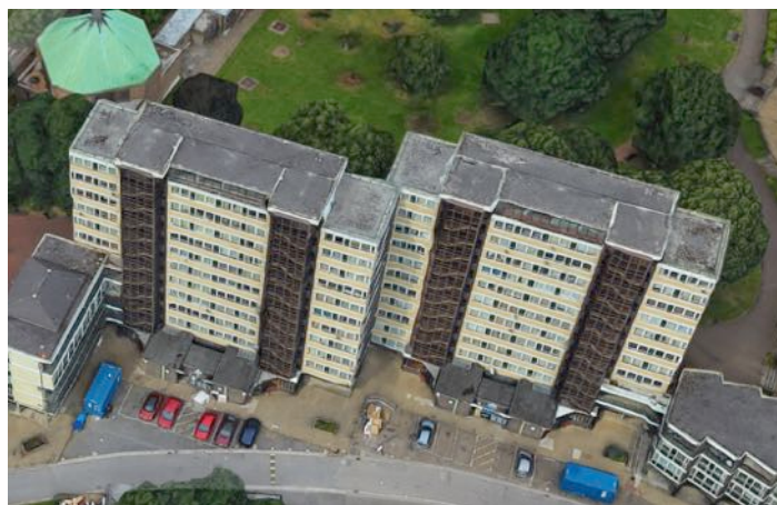
Colechurch House, Tovy House and Proctor House on the Avondale Square Estate appear to have large, unobstructed roof areas suitable for photovoltaic panel installation.
