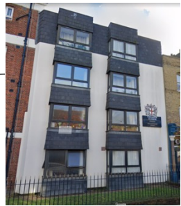
Donnelly House: a 1980s block but with 40% EPCs at D or below. These are potentially heat pump ready with retrofit opportunities to roof, windows and wall.
