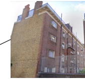
Avondale House : A priority block. Slightly more complex façade but opportunities for window replacements, some wall insulation, roof insulation and PV
