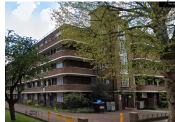
George Elliston House: A priority block. Slightly more complex façade but opportunities for window replacements, some wall insulation, roof insulation and PV
