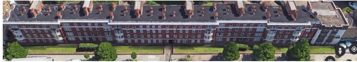
Blake House: a high priority block with a relatively simple but solid brick façade, with retrofit opportunities for the roofs and windows.
